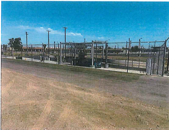
After – Trash Screen & Diversion Structure
